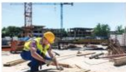
Sites de construction
